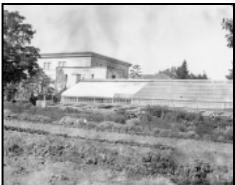
The 1924 Lord & Burnham greenhouse, and experimental gardens where the current parking lot is located, 1933. Photograph by Nicholas Valle. Barnes Foundation Archives.
